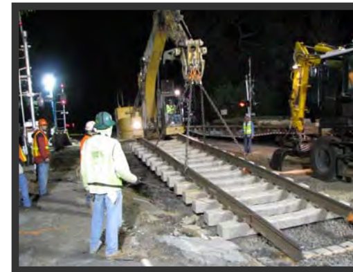
Removing Concrete Panels
