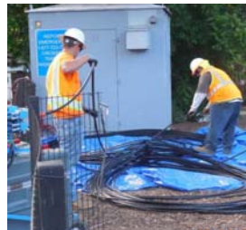
Preparing to install fiber
