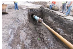
Boring (required at many crossings, within the Caltrain right of way)
