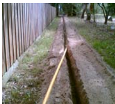
Trench (42" deep x 9.5" wide, within the Caltrain right of way)
