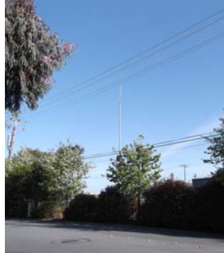
Example 80' pole already on right of way
