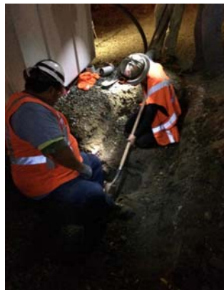
Hand Trenching near a Signal House
