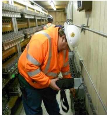
Performing end of work ground verification test
