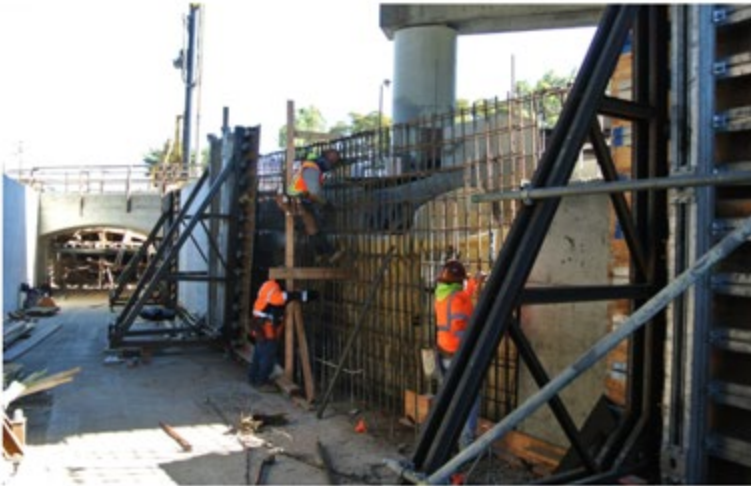
Ramp 3 Construction (West Station Access)
