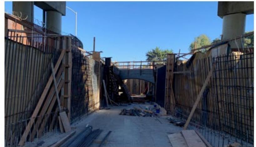
Construction of West Station Access
