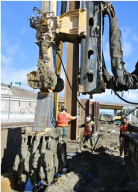
Ramp 1 Construction – Shoring (East Station Access)
