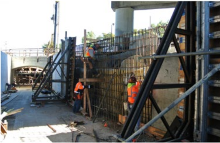
Ramp 3 Construction (West Station Access)
