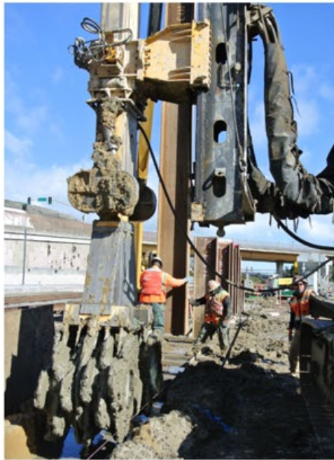
Ramp 1 Construction – Shoring (East Station Access)
