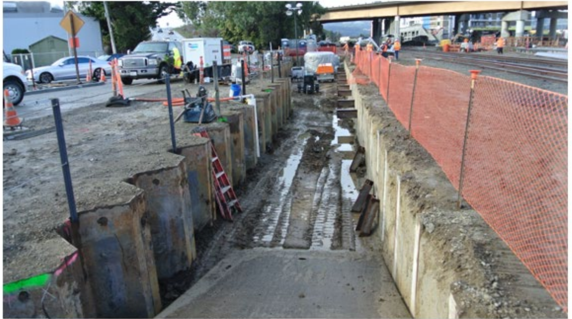
Ramp 1 Construction – Shoring (East Station Access)
