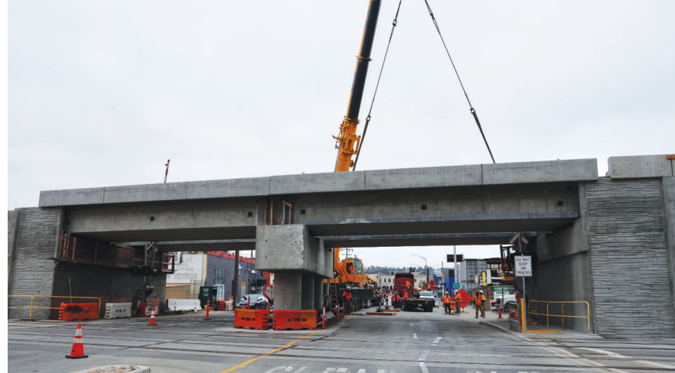
Rail bridge will allow trains to skip traffic @ 25 th Avenue
