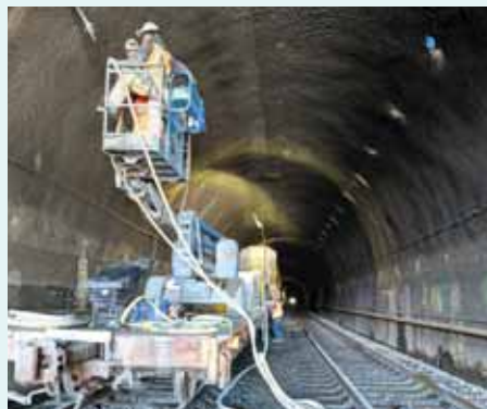
Caltrain Electrification Tunnel Work
