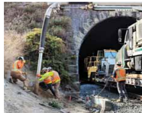
Workers get tunnels ready for electrified service.
