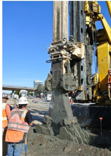
Ramp 1 Construction – Shoring (East Station Access)
