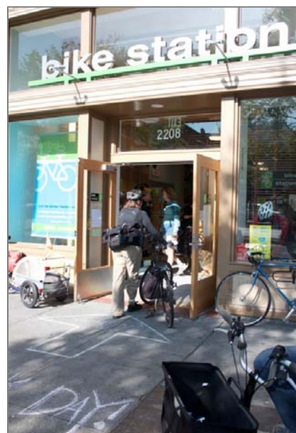
Image 9 - Staffed parking facilities offer high security to customers
