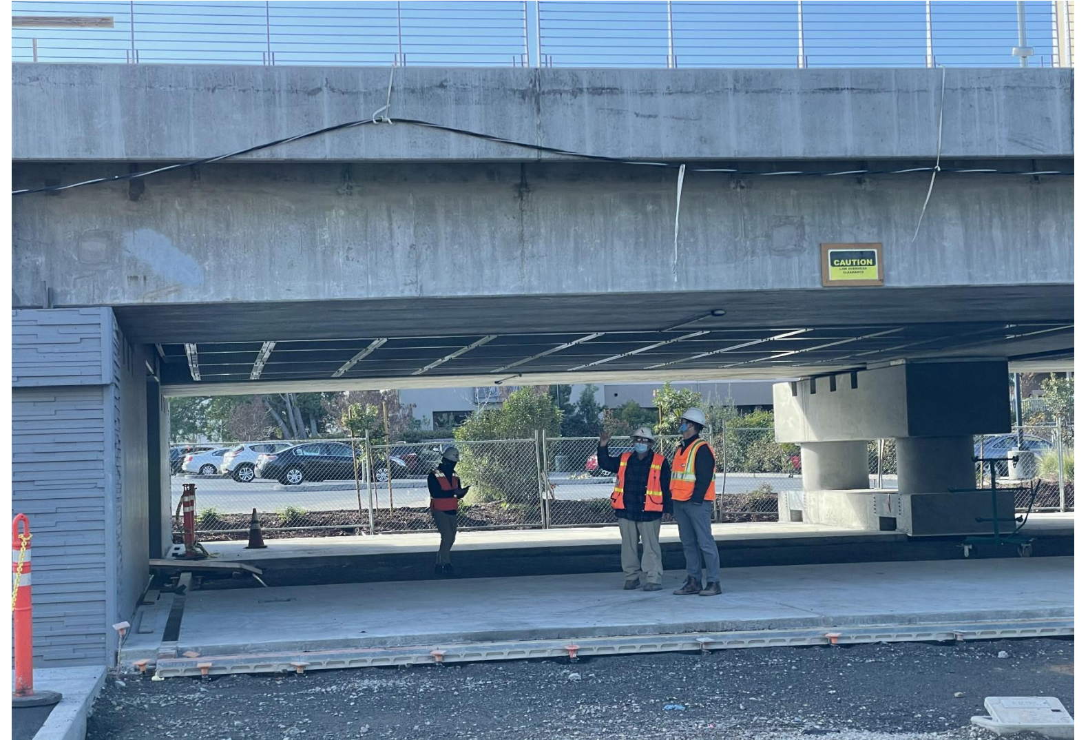
Pedestrian Underpass Bridge
