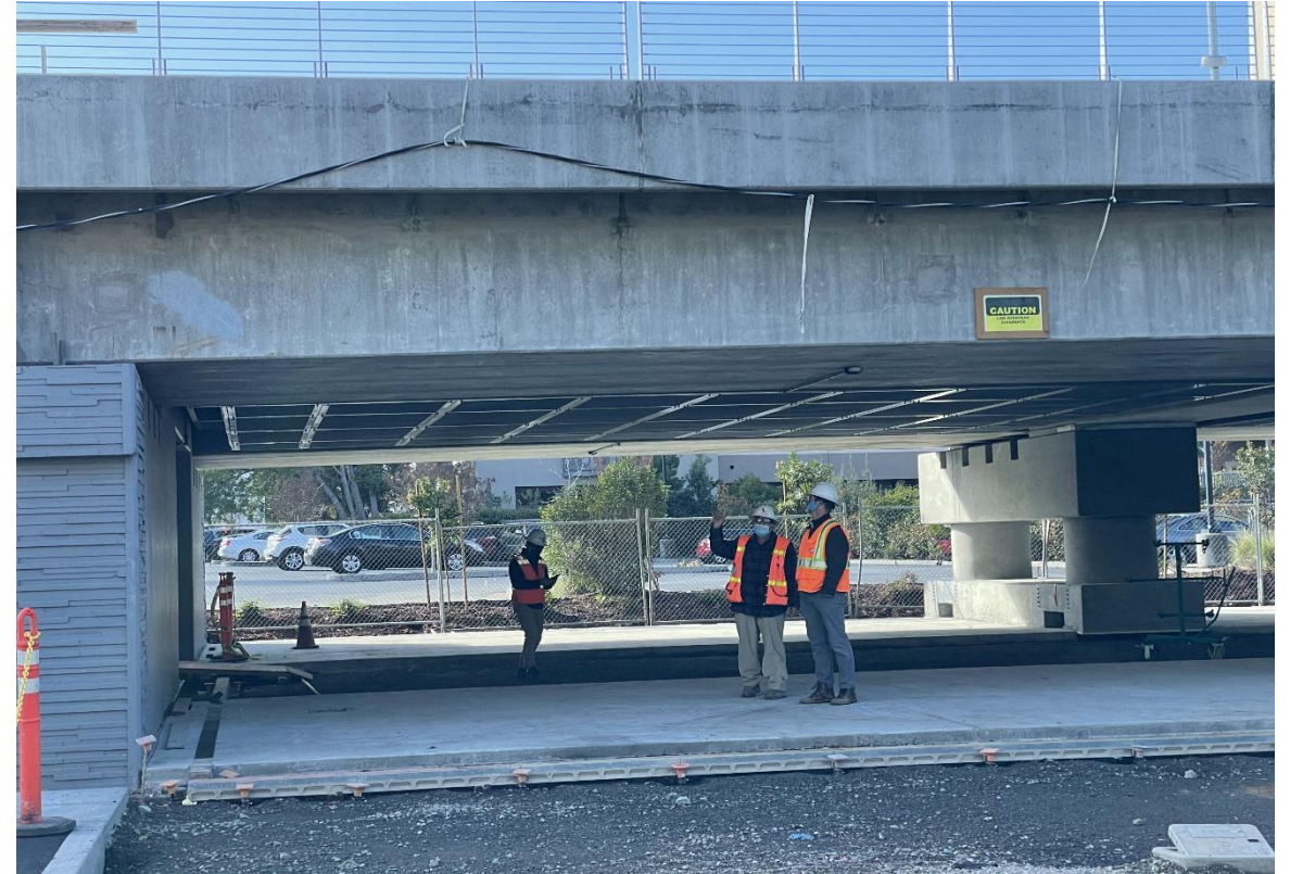
Pedestrian Underpass Bridge
