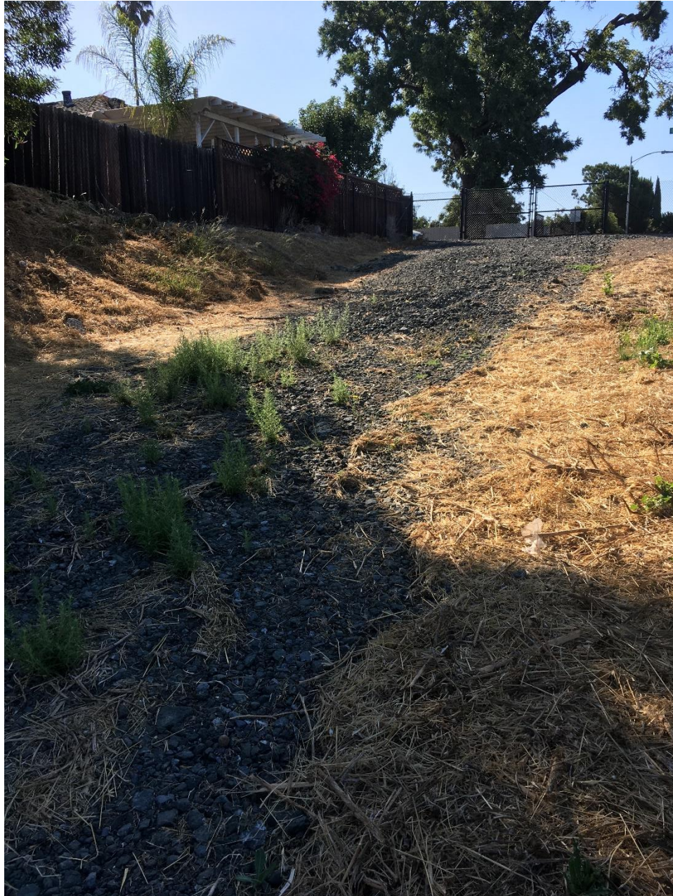
Photo 6. Gravel access road for flood control basin. This area was mapped as developed habitat.
