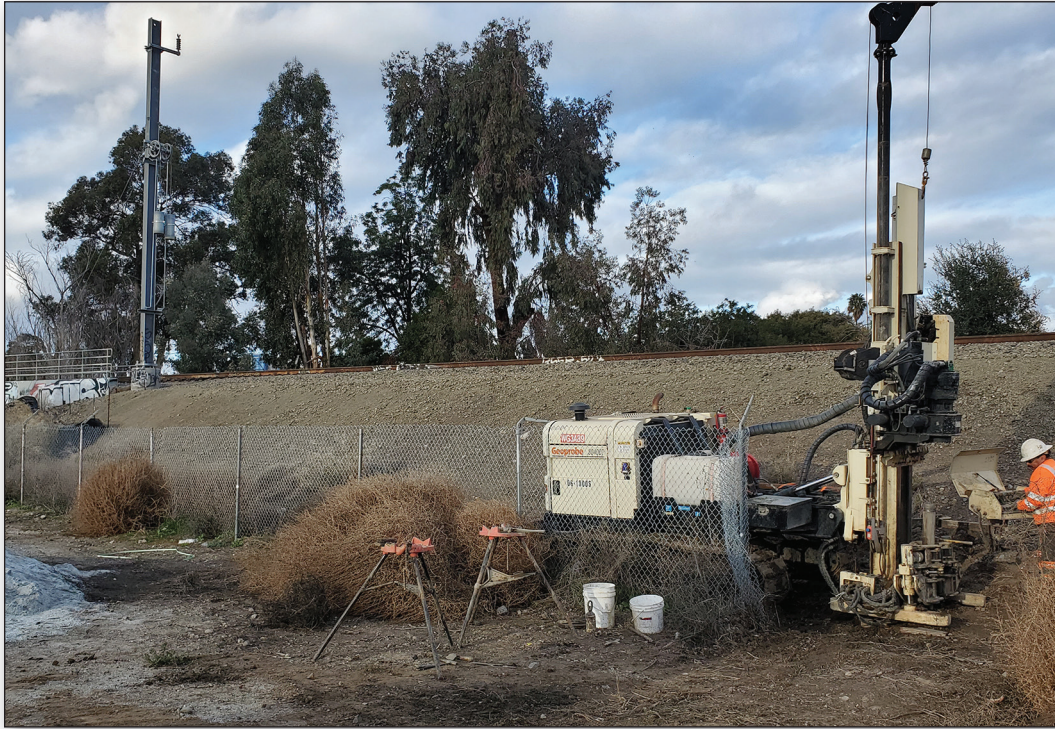
Drilling Core 2, view to the north.
