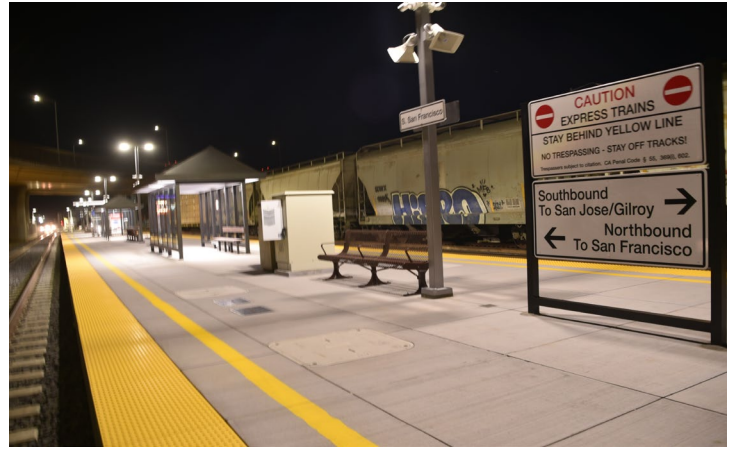
Photo 2 - New platform signage
