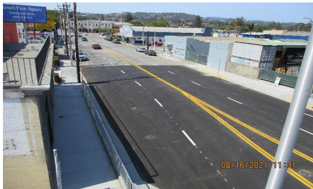
Photo 4 - 25th Ave. Opening
