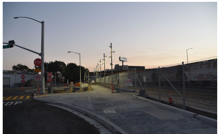
Photo 4 - Poletti way looking towards East Plaza
