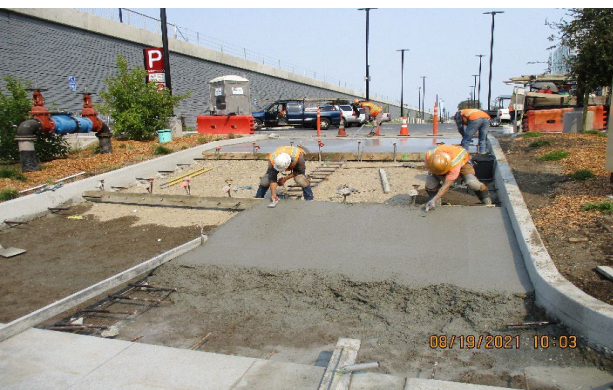
Photo 3 - New Driveway for Bike Path
