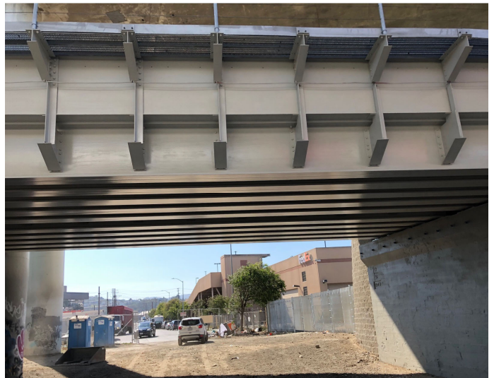
Photo 4 - New Napoleon Bridge
