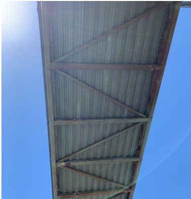
Photo 2 - Pedestrian bridge (underside)
