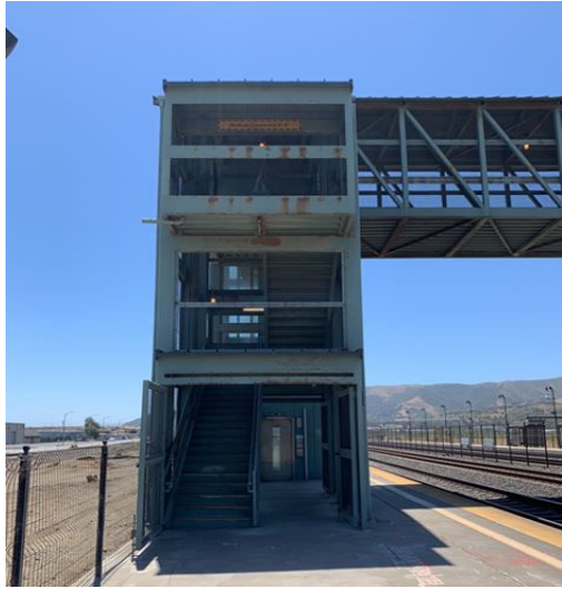
Photo 4 - Stair Case (east side)
