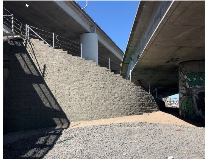
Photo 2 - Napoleon Northeast Retaining Wall
