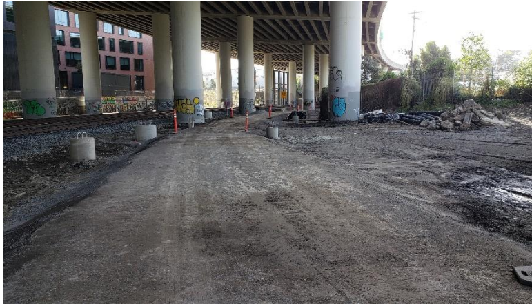
PS-1 – Access road build up and grading
