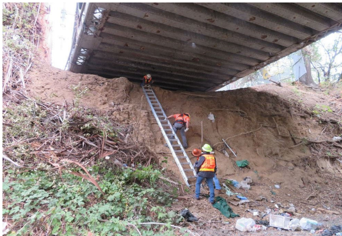
Photo 3 - Inspection crew setting ladder via north side
