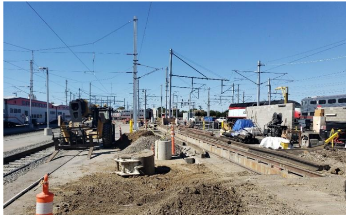
Construction of the North and South Pit Extension
