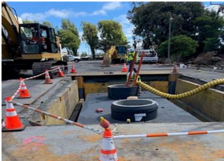
Installation of the vault at the Healthpeak Property
