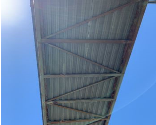
Photo 2 - Pedestrian bridge (underside)
