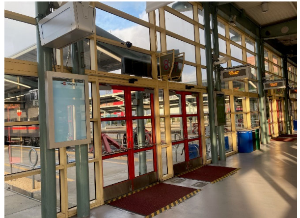
Photo 4 - Doors 5, 6, 7 and 8 APC
