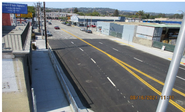
Photo 4 - 25th Ave. Opening
