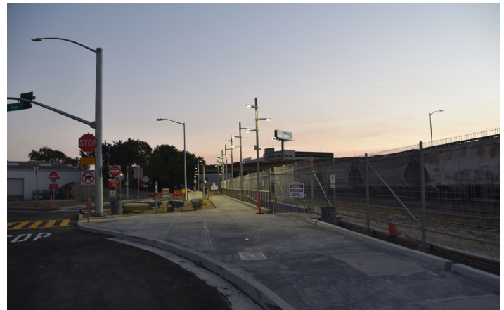
Photo 4 - Poletti way looking towards East Plaza
