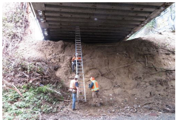
Photo 4 - Inspection crew via north side abutment
