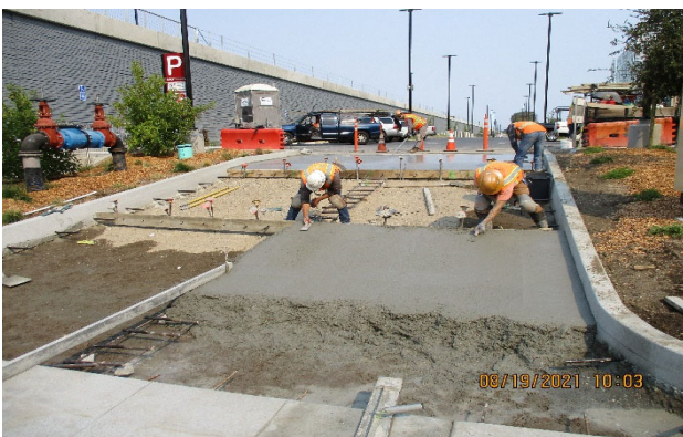
Photo 3 - New Driveway for Bike Path
