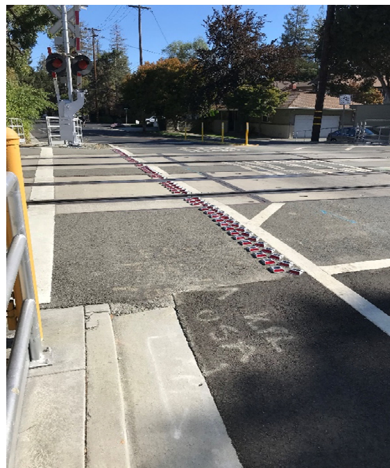
Photo 2 - New LED pavement markers at Glenwood Ave in Menlo Park
