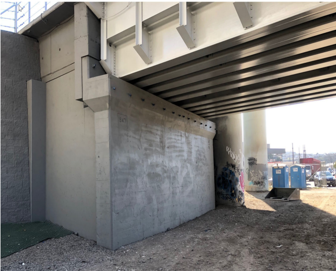
Photo 3 - Napoleon South Abutment
