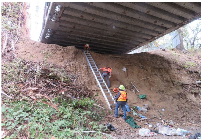
Photo 3 - Inspection crew setting ladder via north side
