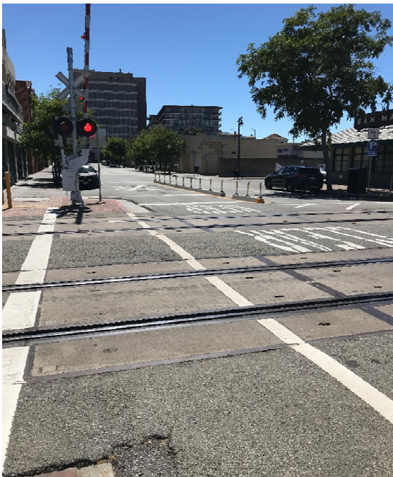
Photo 1 - New median on 1st Ave in San Mateo
