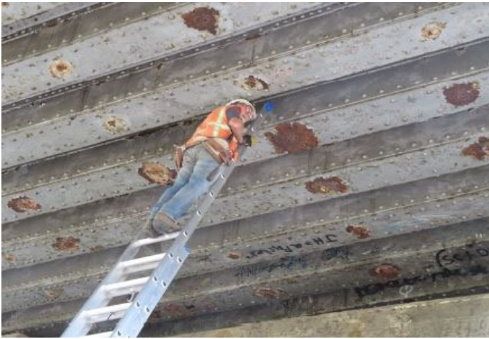
Photo 1 - Inspection crews via underside of bridge via south side
