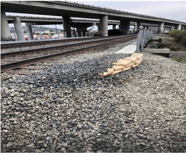
Photo 1 - Marin Street New Walkways
