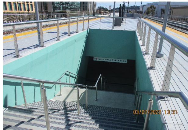
Photo 4 - Stairs Paint Touchup at Hillsdale Station
