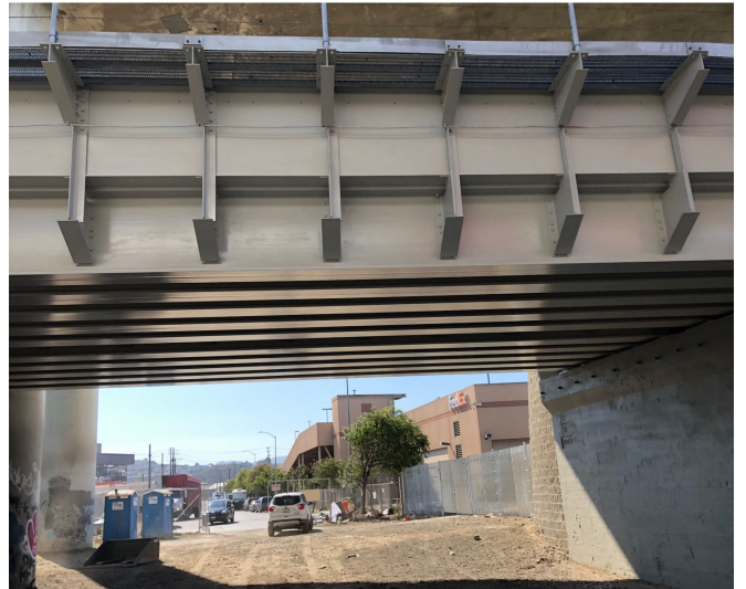
Photo 4 - New Napoleon Bridge
