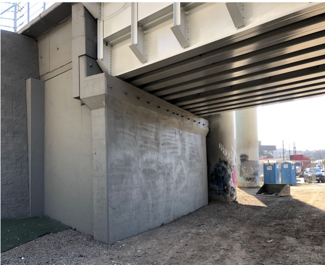
Photo 3 - Napoleon South Abutment
