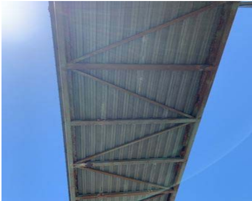
Photo 2 - Pedestrian bridge (underside)
