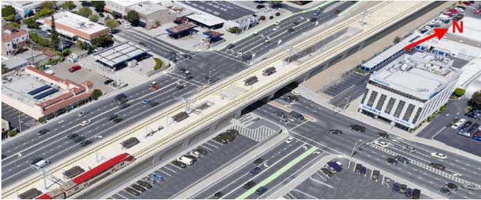
Photo 1 - After construction (rendering)
