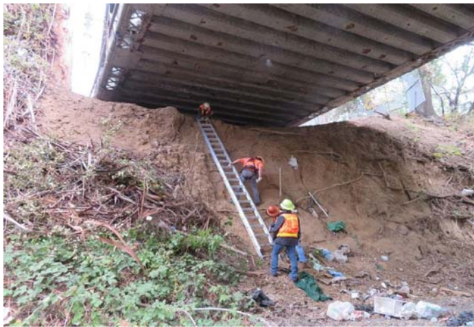
Photo 3 - Inspection crew setting ladder via north side
