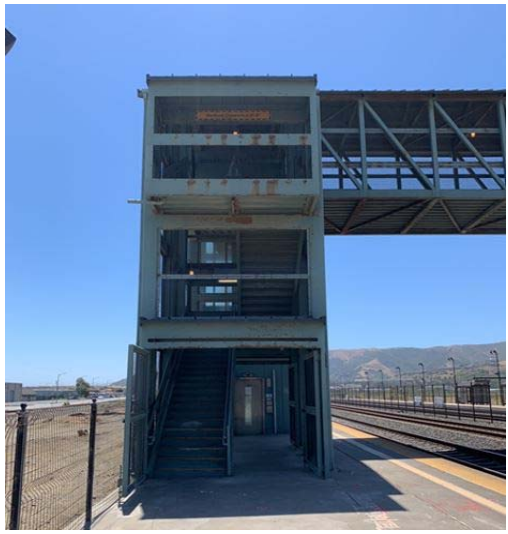
Photo 4 - Stair Case (east side)
