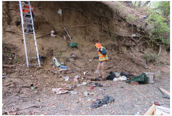
Photo 2 - Inspection crew cleaning up debris
