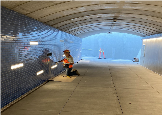
Photo 3 - Ped Underpass looking east
