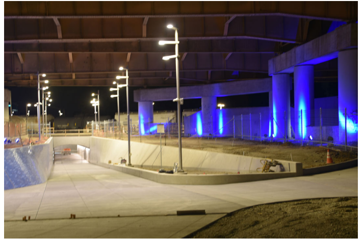
Photo 4 - Poletti Way looking towards East Plaza
