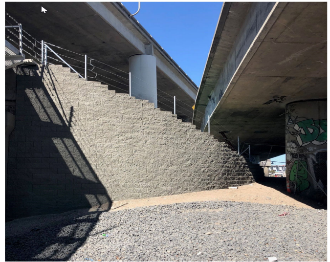
Photo 2 - Napoleon Northeast Retaining Wall
