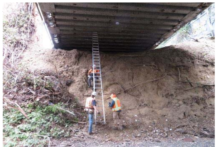
Photo 4 - Inspection crew via north side abutment
