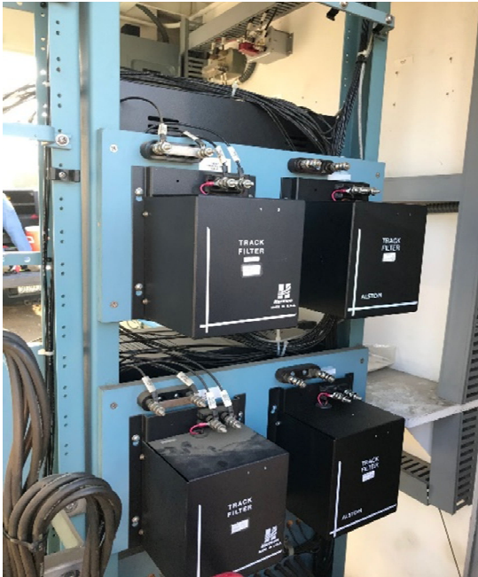
Photo 1 - New advance signal preemption equipment
