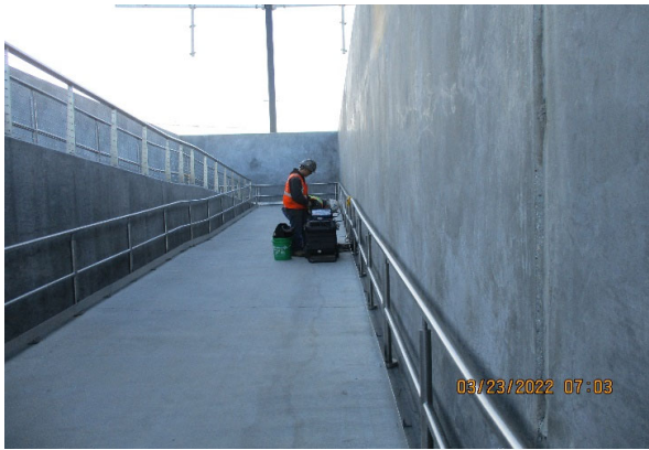
Photo 3 - South Ramp fixing plate kickers
