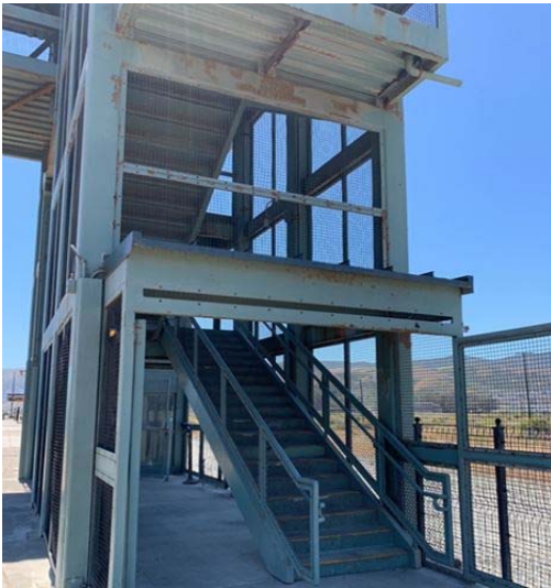
Photo 3 - Stair Case (west side)
