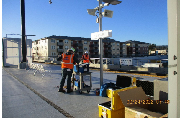
Photo 2 - OCS Grounding Testing.
