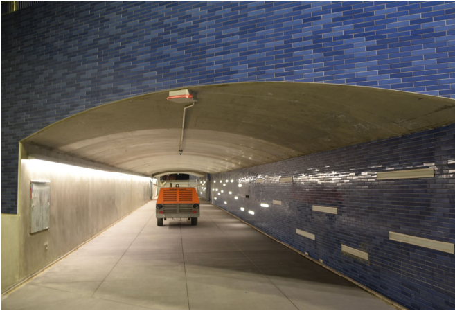
Photo 1 - Ped tunnel looking west
