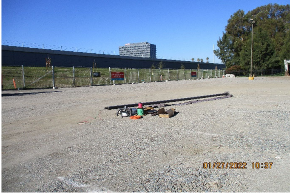
Photo 1 - 25th N Yard Lighting Pole
