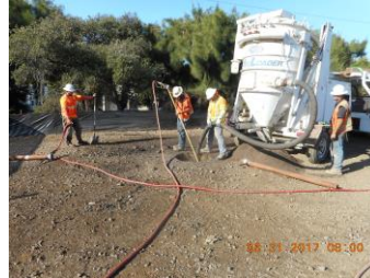
Test pile installation in preparation for foundation installations
