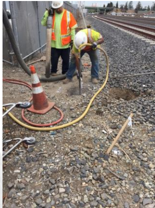
Potholing – to identify utilities
