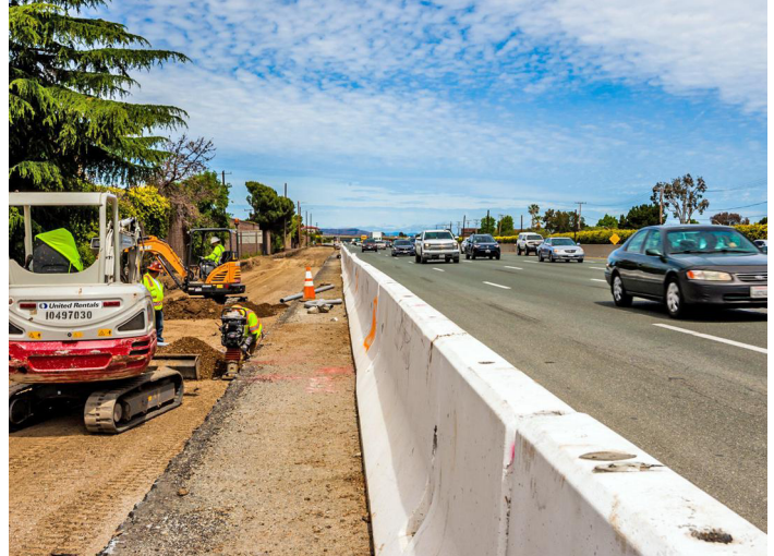
Photo: US-101 Express Lanes Construction
