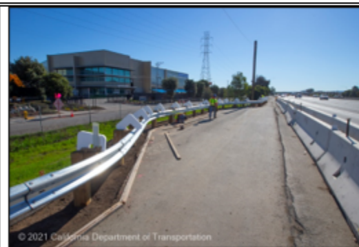
A new maintenance vehicle pullout area in the shoulder
