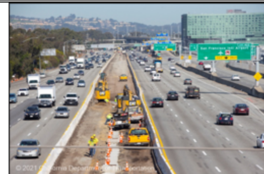
Construction crews excavating in the median
