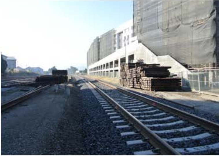
New MT2 Track – Looking South
