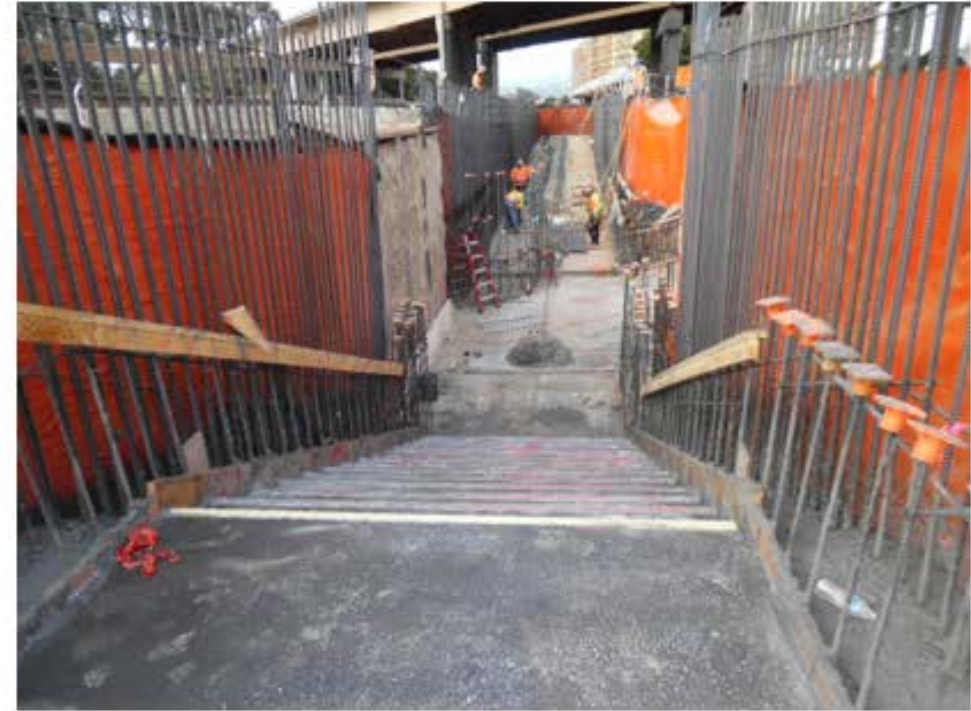
Construction of Ramp 2 Access to Platform
