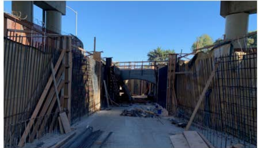
Construction of West Station Access
