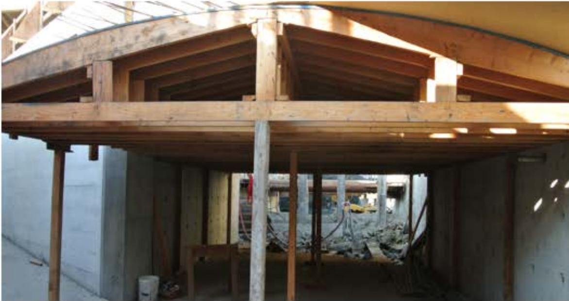
Arch Formwork to Platform and Underpass
