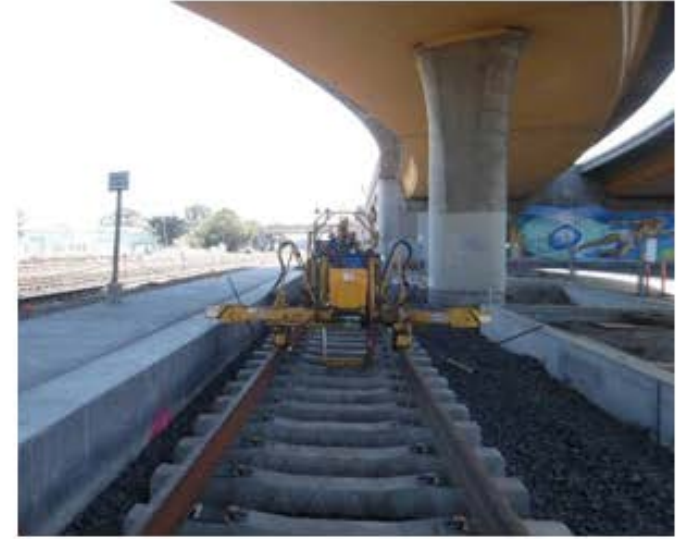
New MT2 Track – At Center Platform
