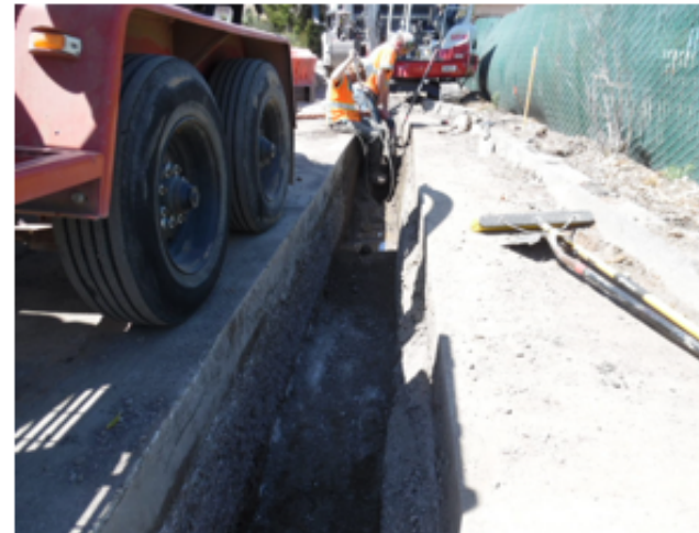
Utility Relocation – UP Joint Fiber Optic Trench (August 2020)
