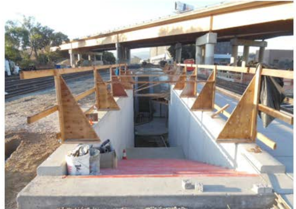
Stair 2 Access to Platform
