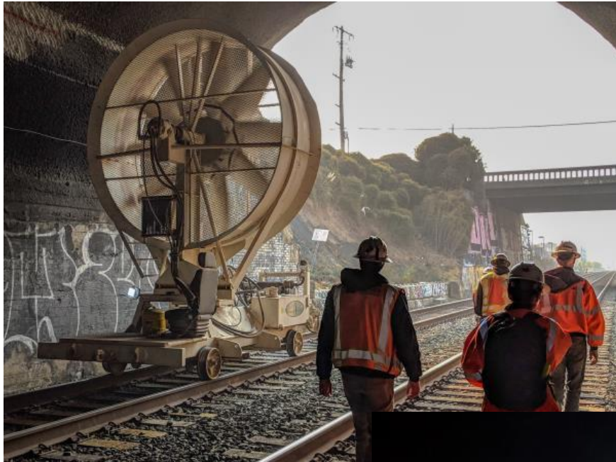
Fan used to maintain airflow during notching
