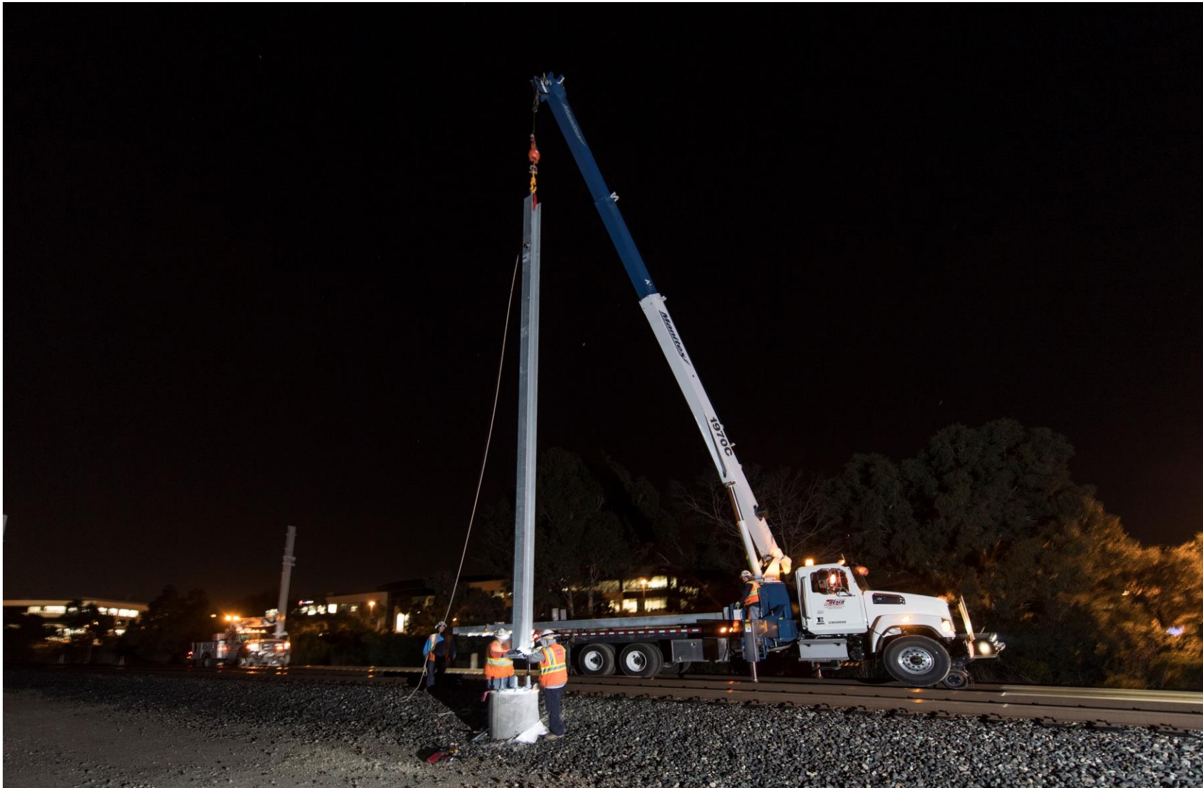
OCS pole lifted off flatbed truck
