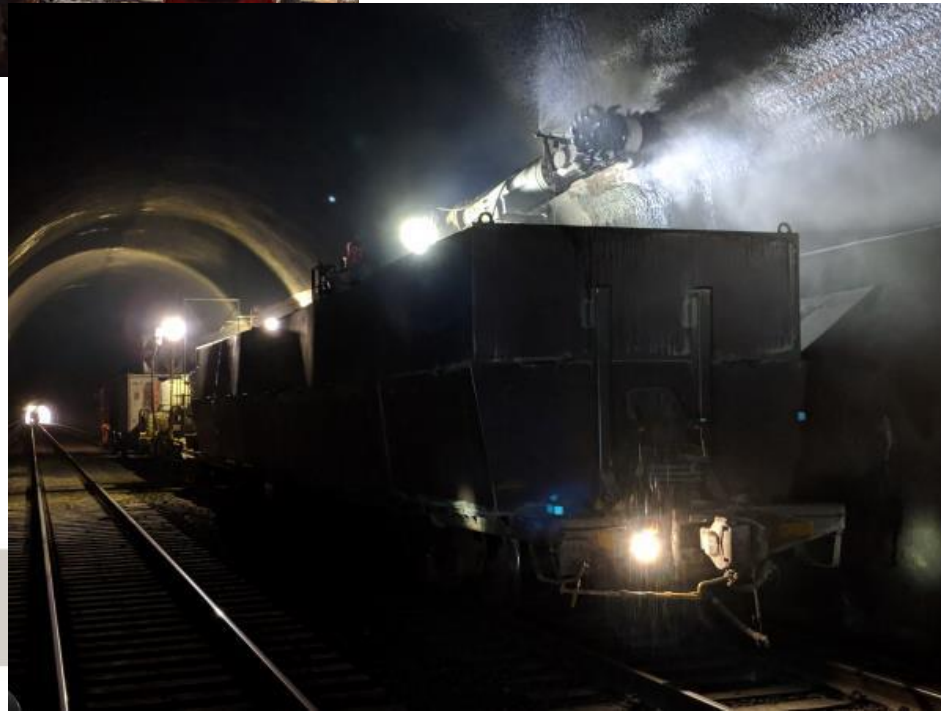
Roadheader Notching Operation
