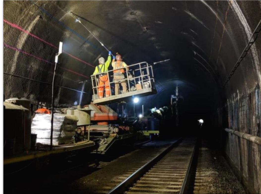
Rock Bolt Installation (foreground) Grout Hole Drilling (background)
