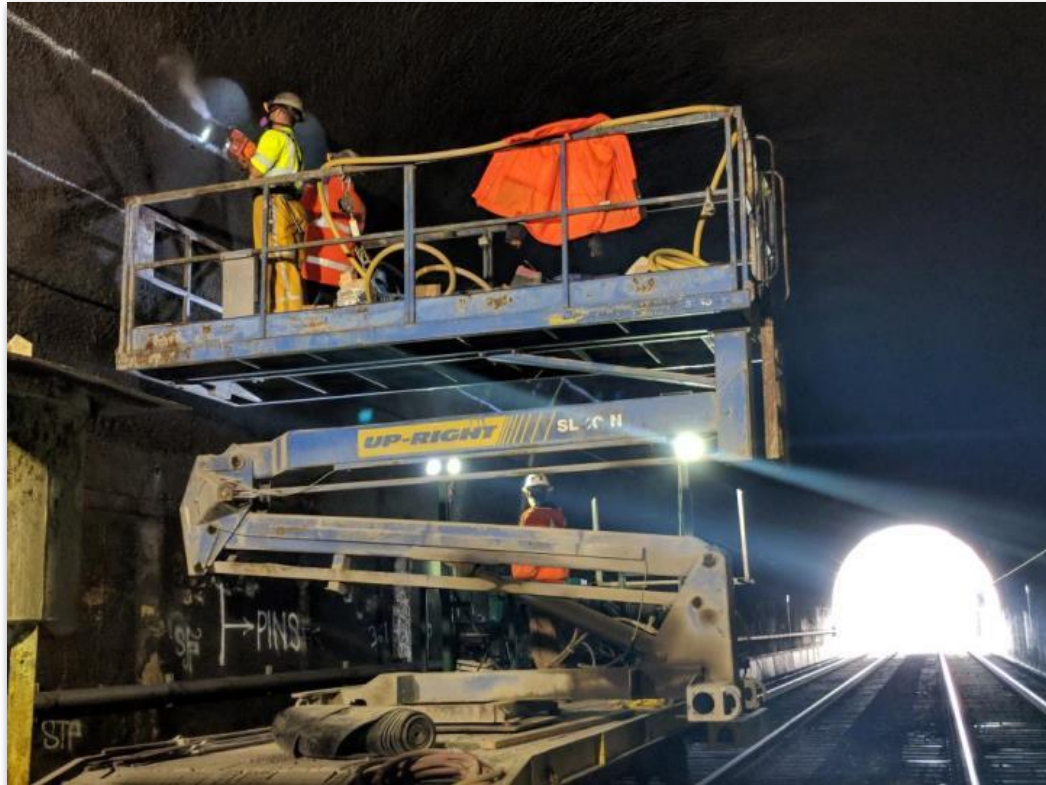
Dry Fix Pin Installation
