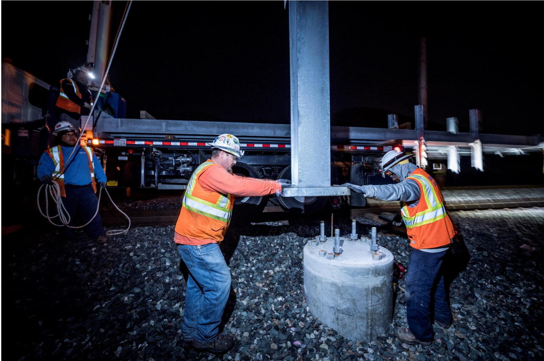
Crew placing OCS pole on foundation
