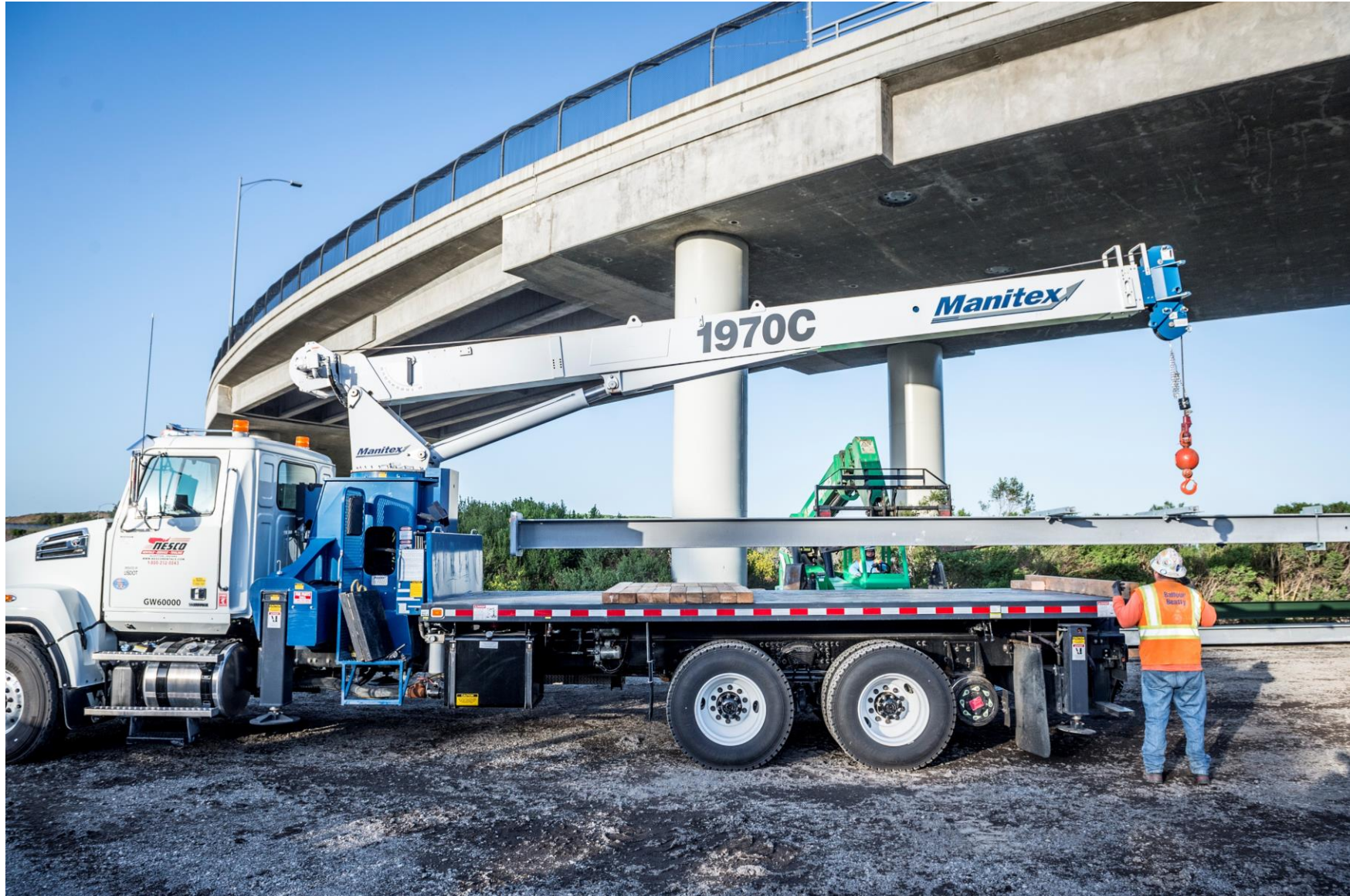
OCS pole on flatbed truck
