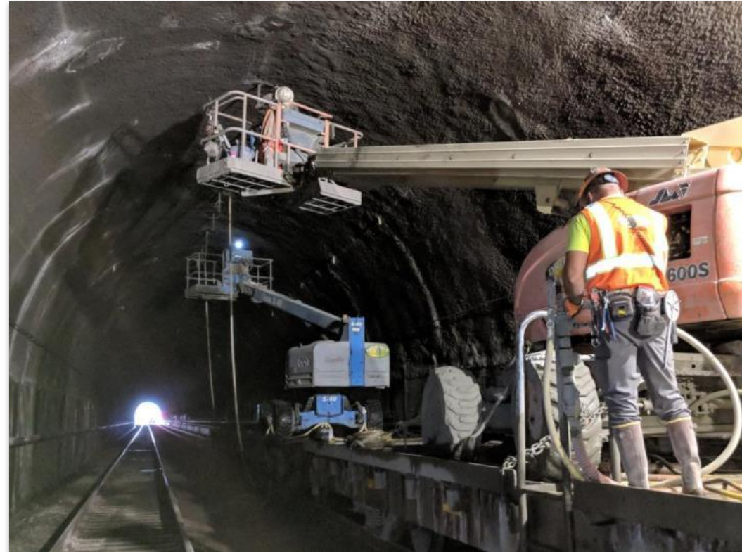
Grouting Operation
