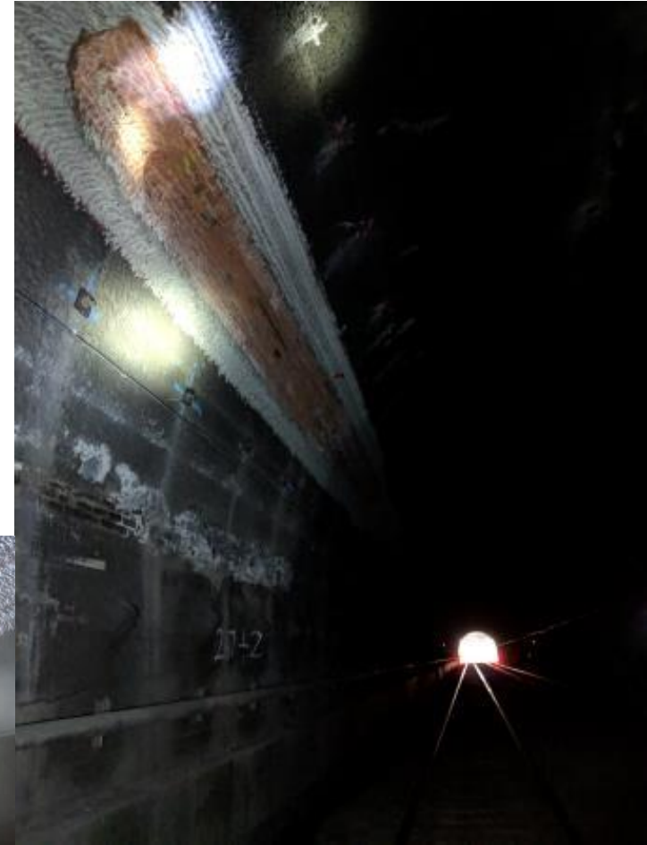
Exposed Brick in Notch
