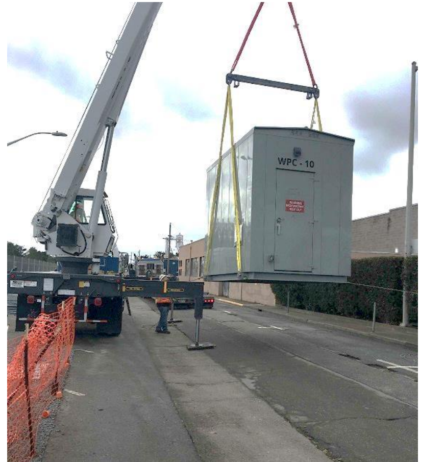
Setting a Wayside Power Cubicle
