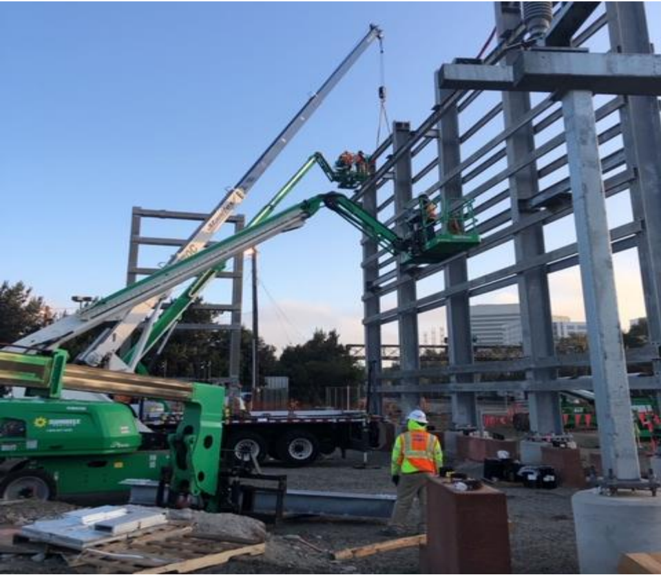
Assembly of Gantry at TPS-1
