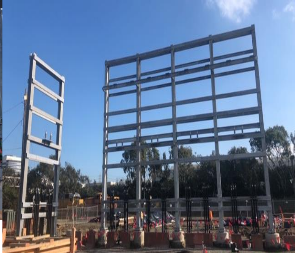
Erected Gantry at TPS-1
