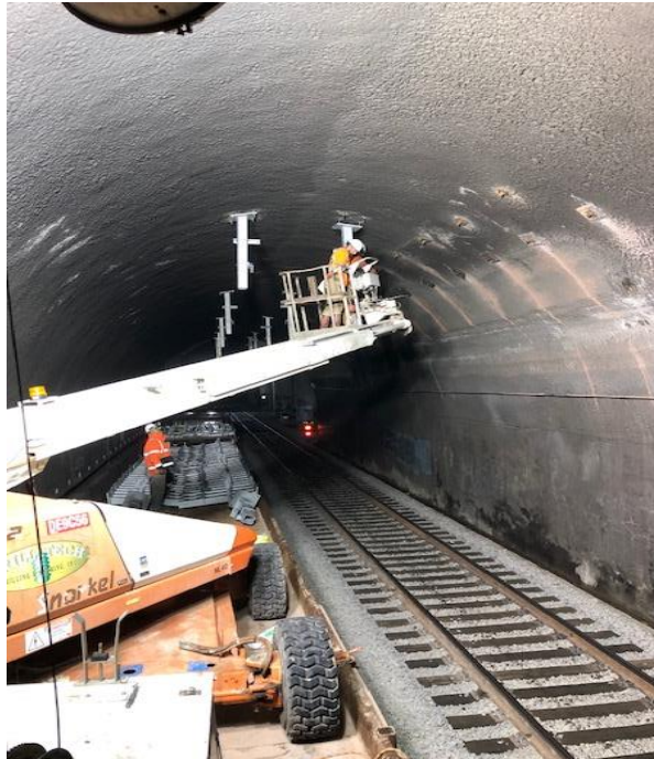
Drop Tube Installation
