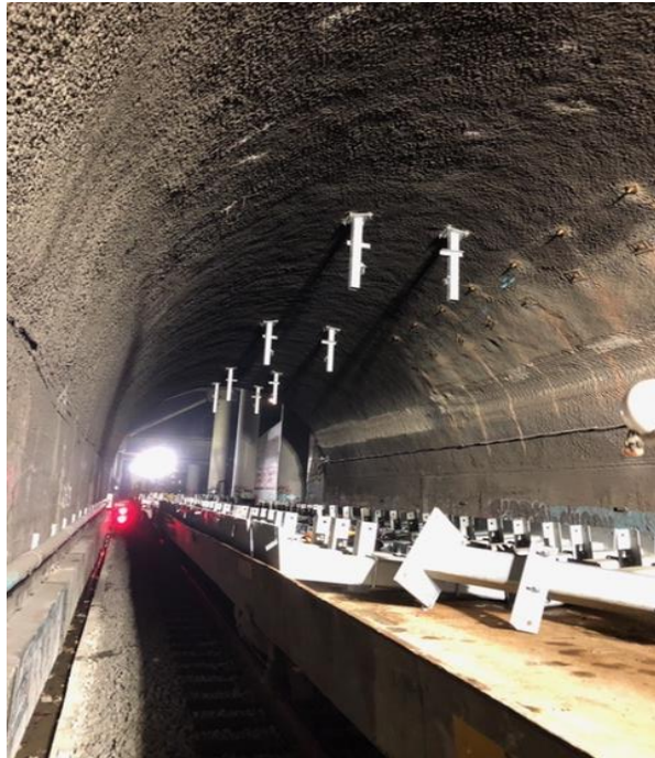
Drop Tube Installation
