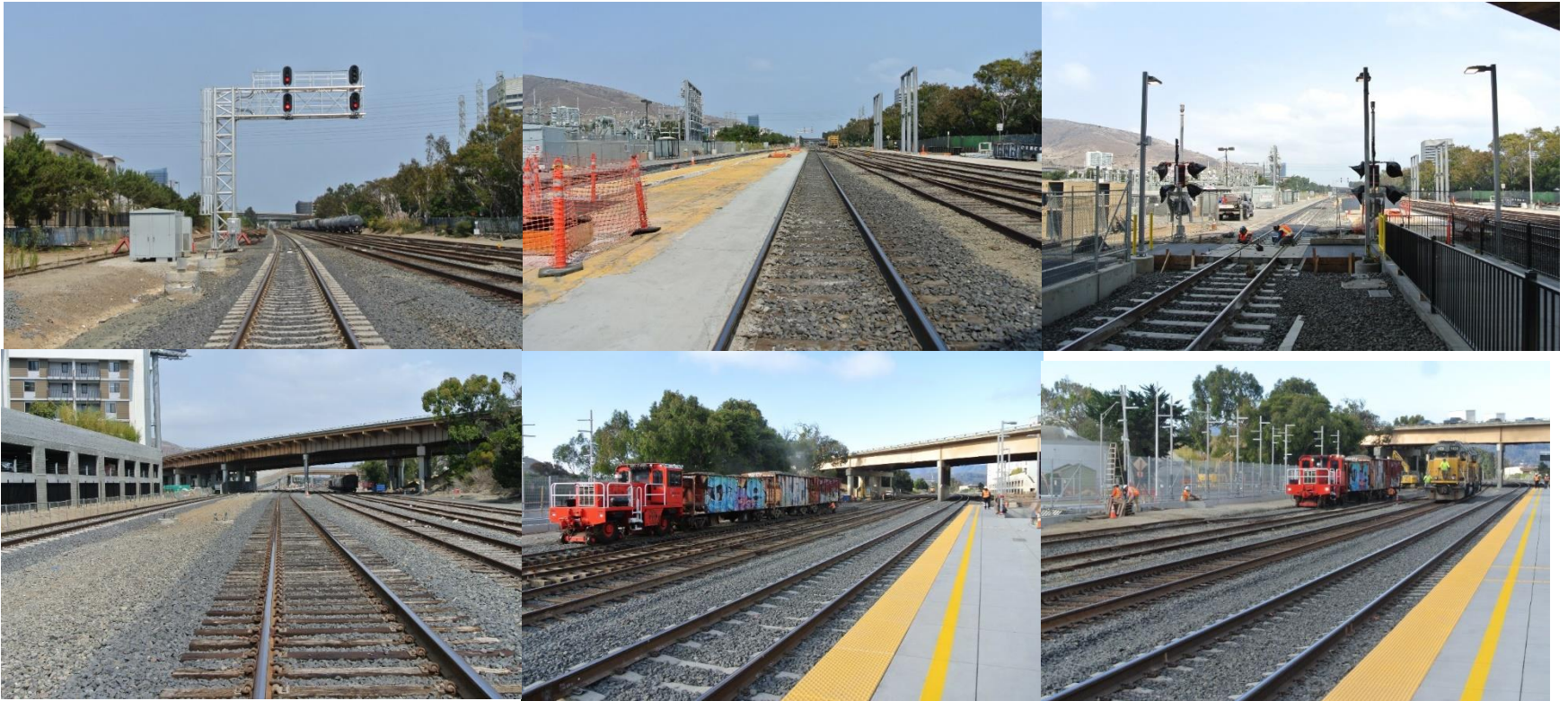
Mainline Tracks & Yard Tracks Work
