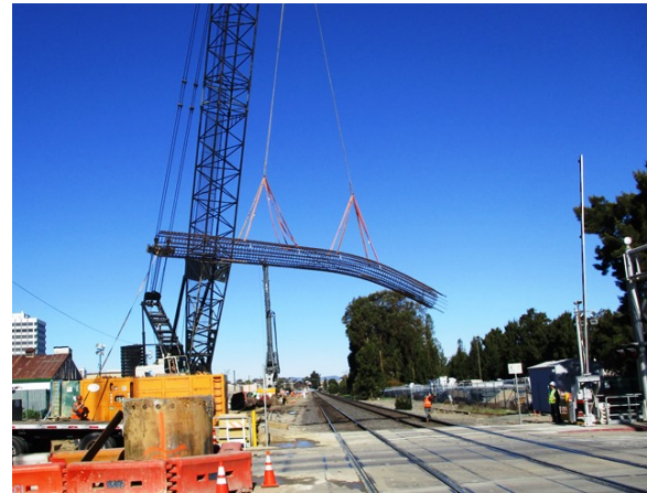
Crane work near 25 th Avenue
