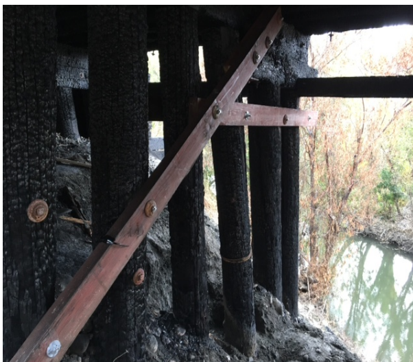
Bridge with new cross bracing installed.
