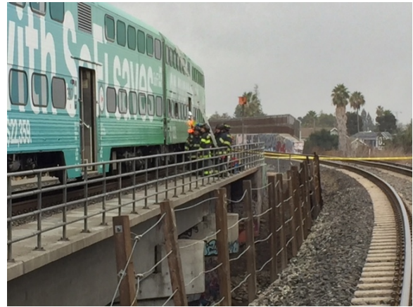
SJFD - Caltrain train on Guadalupe River Bridge
