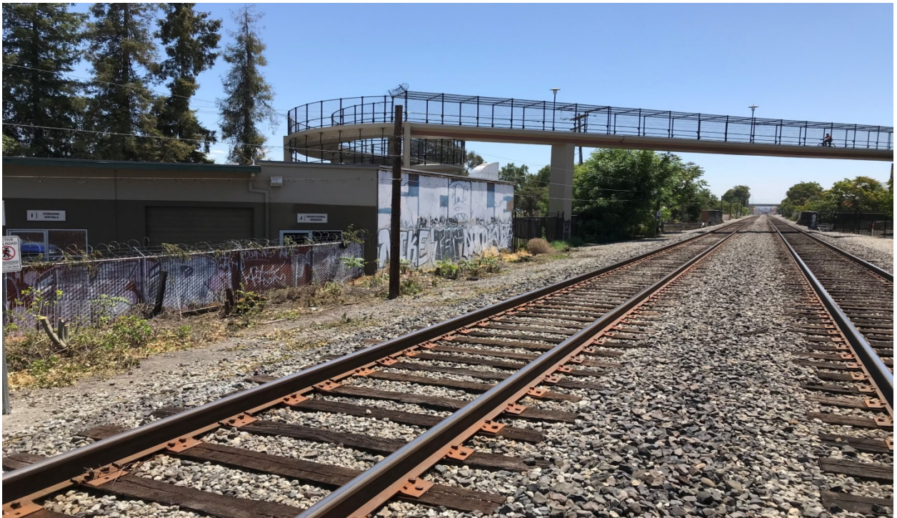
Tree removal at Lafayette Street in Santa Clara - After photo
