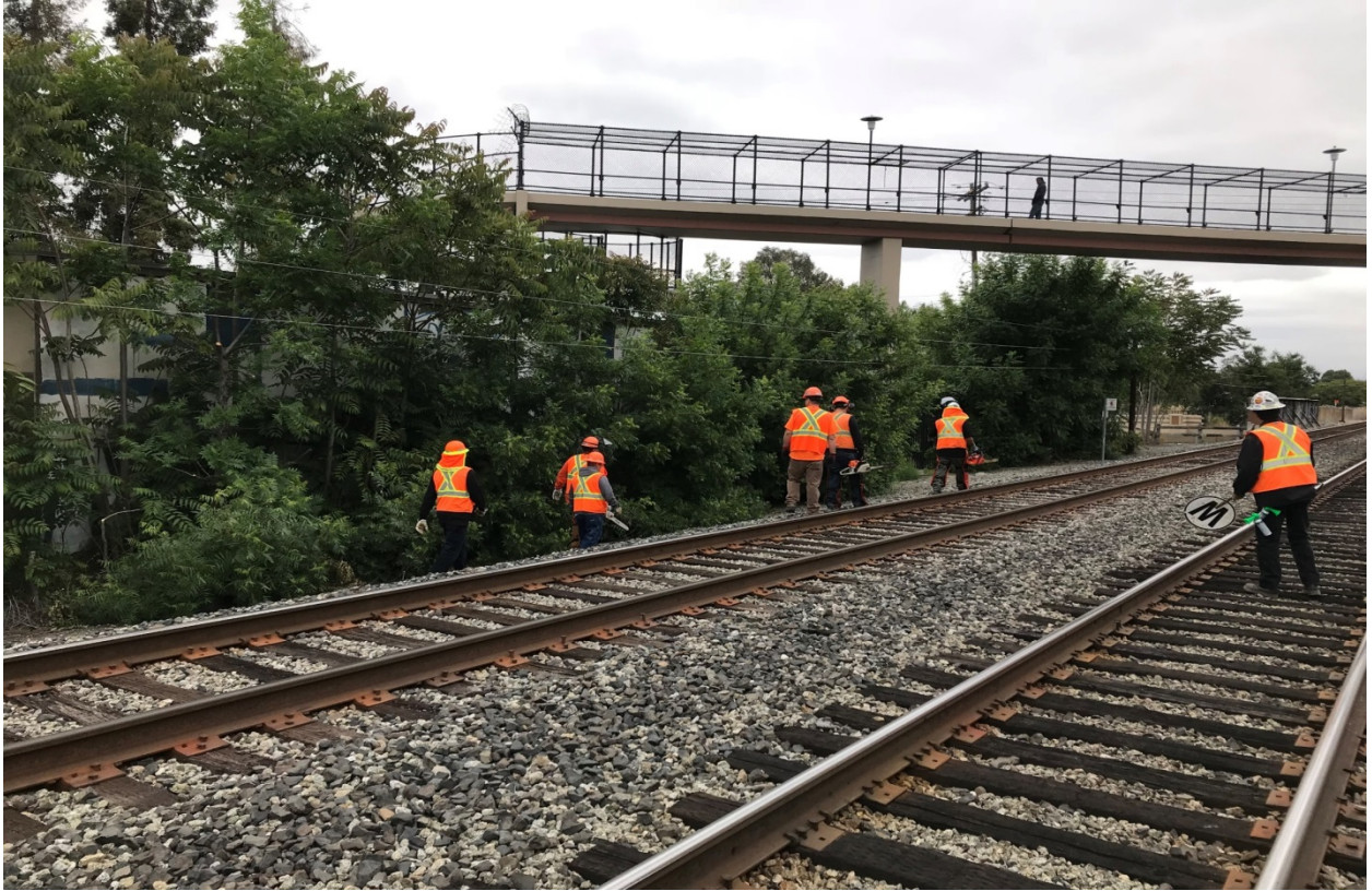
Tree removal at Lafayette Street in Santa Clara - Before photo
