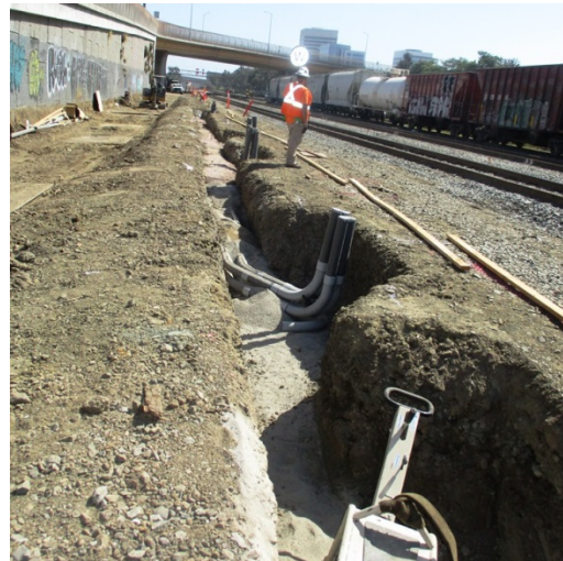
Relocated utility lines
