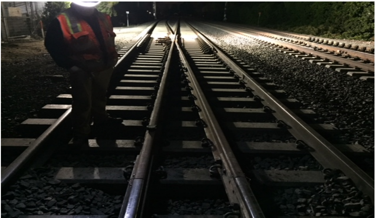
New switch frog installation shown
