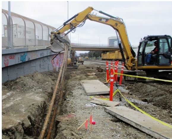
Removal of inactive utility lines
