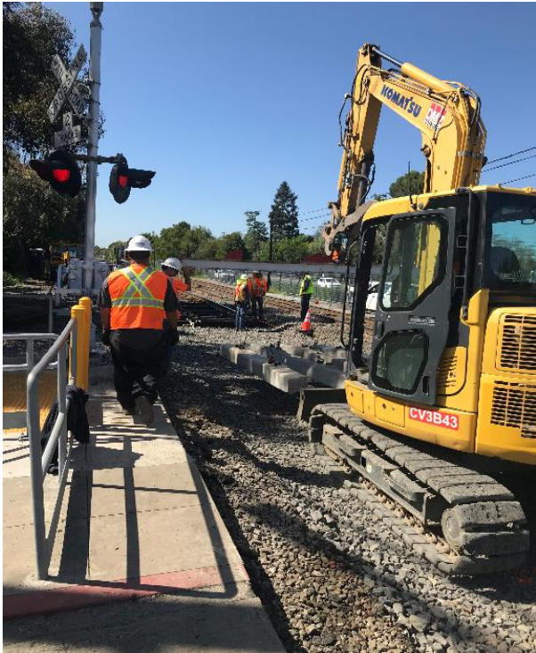
Installation of new ballast, new concrete ties and new rail
