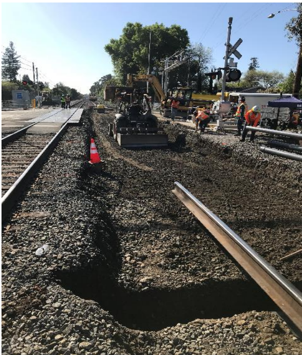
Removal of old ballast and excavation to subgrade. Installation of new underground track drainage pipe and Installation of asphalt layer below future track
