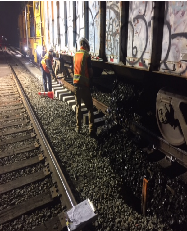
Placement of new ballast over new track and track surfacing
