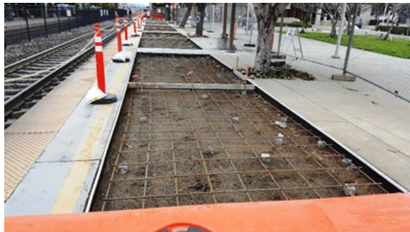
Pavers Removed and Rebar Work Done
