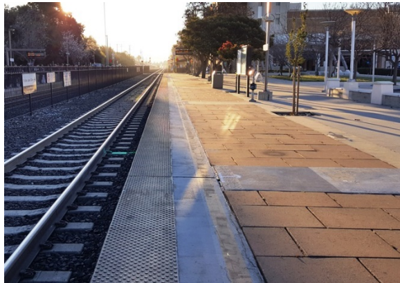
Sunnyvale Station South Bound Platform prior to Construction Work Commencement
