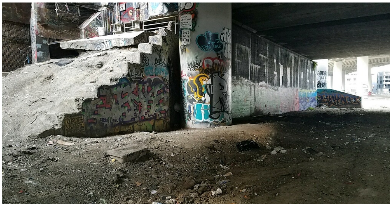
After clean up
