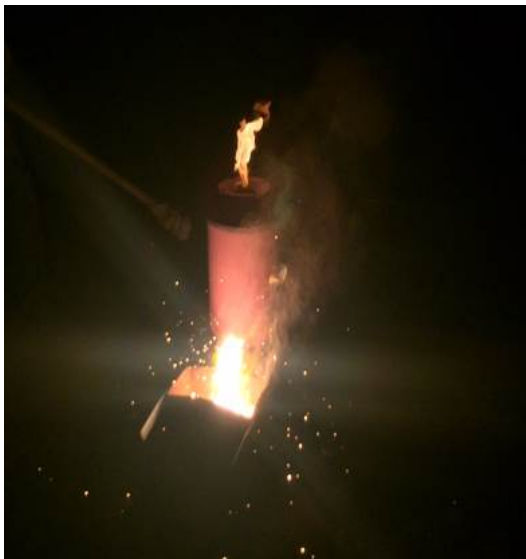
'Shooting' the weld
