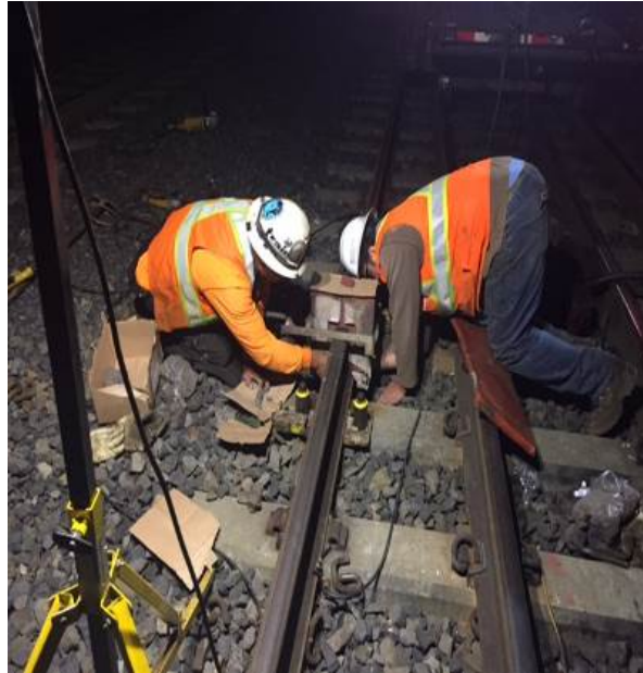
Preparing the rail
