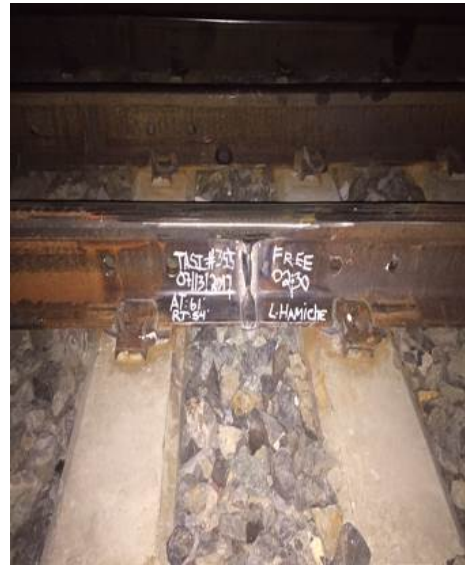
Completed weld
