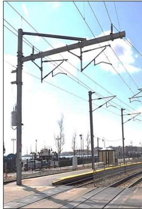
Two Track Cantilever
