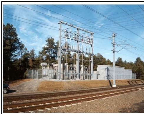
Example Traction Power Substation
