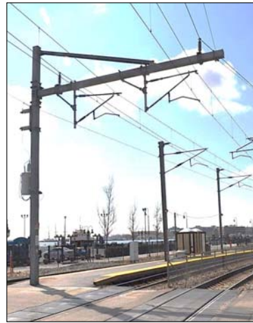
Two Track Cantilever (39)
