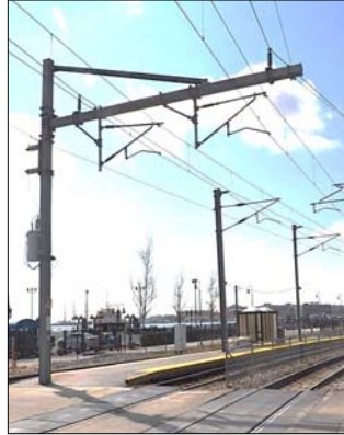
Two Track Cantilever
