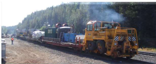
DrillTech on track foundation train
