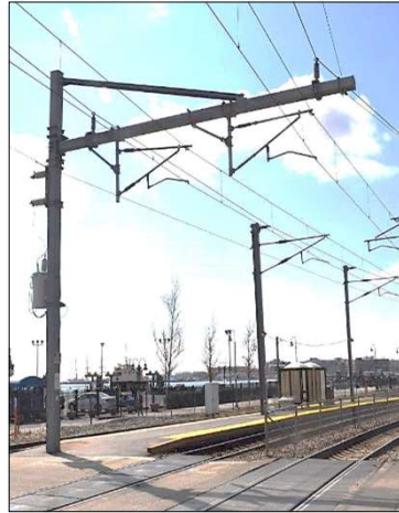
Two Track Cantilever
