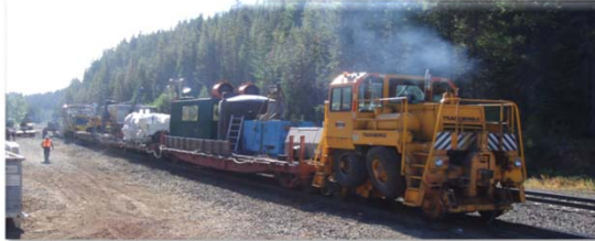
DrillTech on track foundation train
