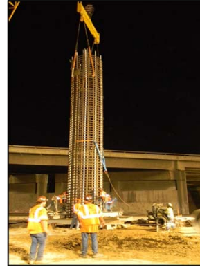
Foundation Rebar Cage
