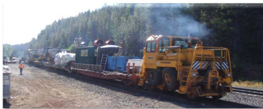
DrillTech on track foundation train
