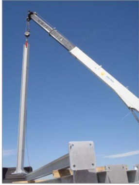
On/off-track crane for installation
