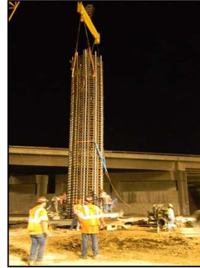
Foundation Rebar Cage
