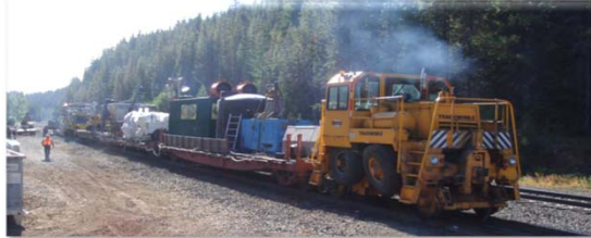
DrillTech on track foundation train
