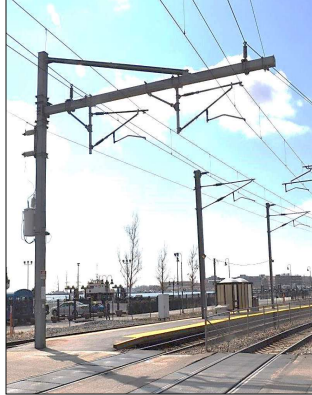
Two Track Cantilever
