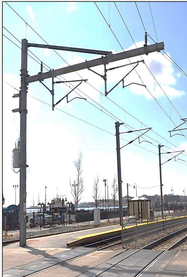
Two Track Cantilever
