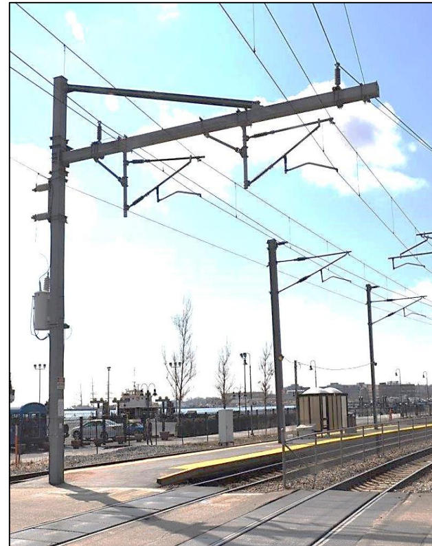
Two Track Cantilever
