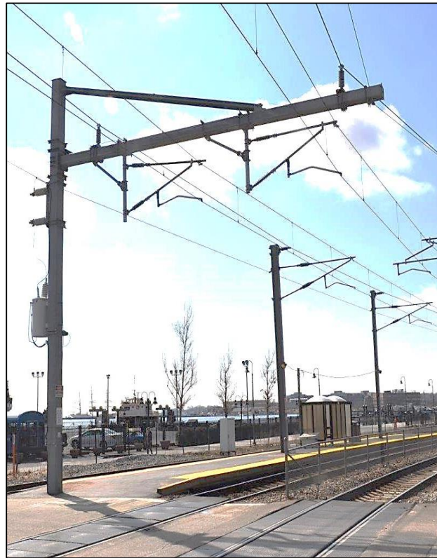
Two Track Cantilever
