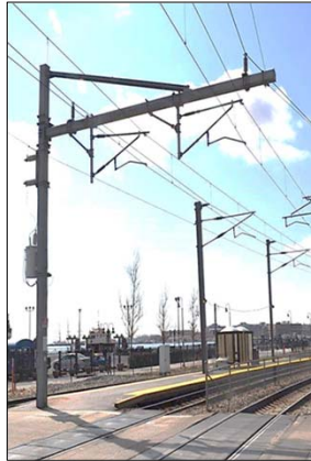
Two Track Cantilever
