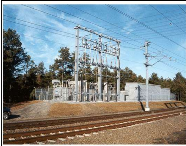
Example Traction Power Substation
