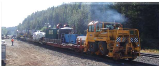
DrillTech on track foundation train
