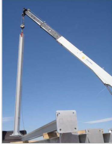
On/off-track crane for installation
